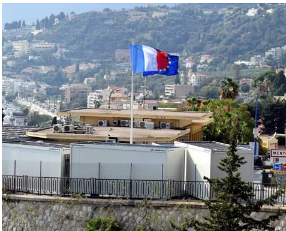
Figure 4: Photo by Nice-Matin 5 showing the prefabricated buildings outside the PAF post at Menton Pont Saint-Louis.
